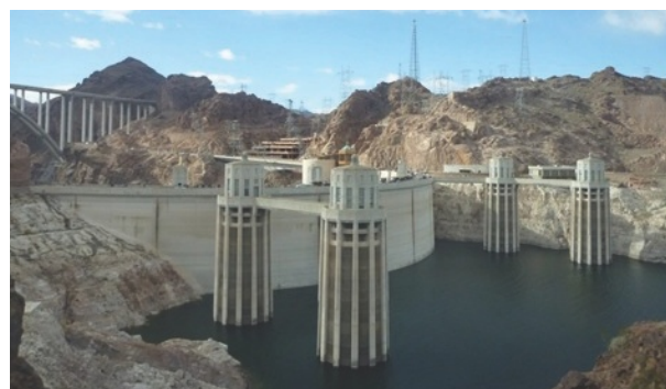
■ Figure 24.2 The Hoover Dam, on the Colorado River, USA, generates about 2000 MW from its hydroelectric turbines
